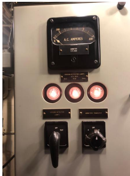
Figure 14: Ground detection lamps on USS Slater (DE-766) (photo by Norbert Doerry)
